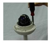
Attach the camera to the pendant mount using the machine screws
