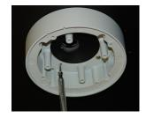
Use the dry wall anchors and machine screws to mount the junction box and rubber gasket to the wall.
